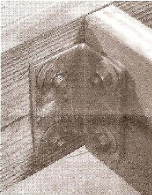
17. Attach inside stringers with angles and washer plates. Do not tighten.
