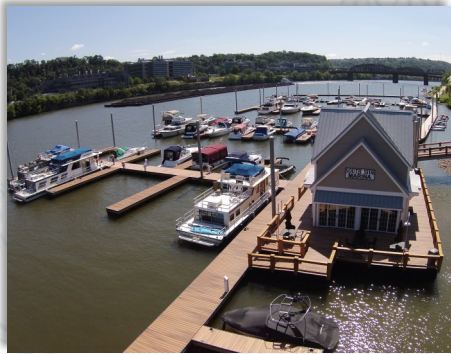
2 Story, Marina Offices, Restrooms, & Vending
