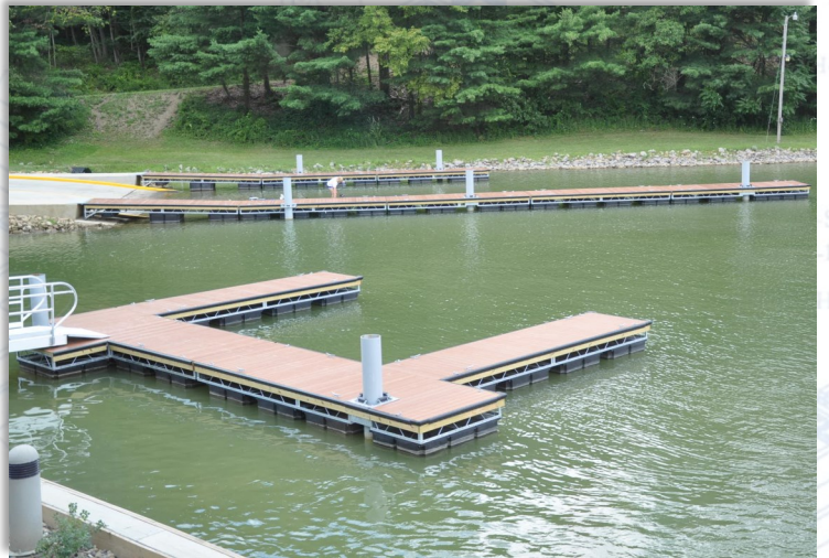
Watershed Conservancy Launch docks in Ohio
