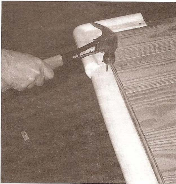
28. Nail down rubrail – use stainless nails (B-RN). We recommend a nail every 6" top and bottom.
