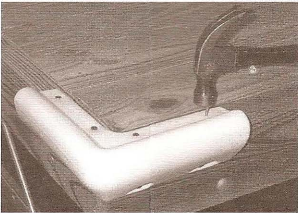
27. Nail vinyl corners (RR-CB) with stainless nails (B-RN).
