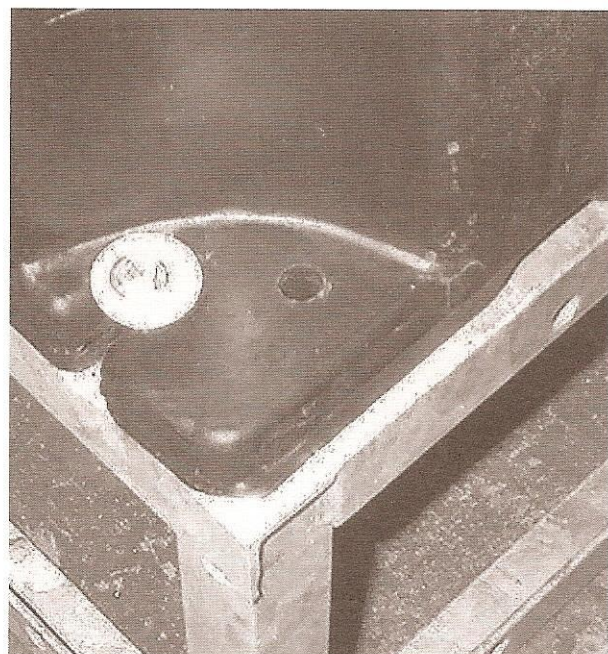
9. Use \frac{3}{8} " hex head socket to fasten drums securely to truss frames.
